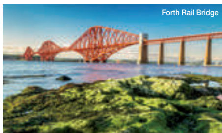
Forth Rail Bridge
